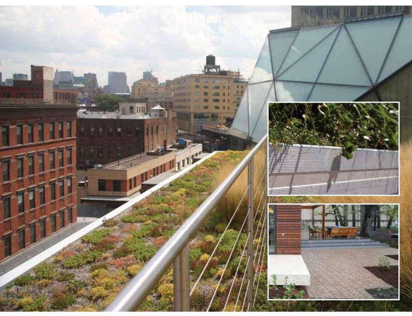
GeoEdge<sup>TM</sup> is a flexible, multi-height, durable aluminum edge restraint and component system for the green build environment, including landscaped roof systems and permeable pavement applications. GeoEdge has a sturdy L-shaped profile available in several heights, with a choice of a solid wall or a slotted wall, which allows for water runoff.
